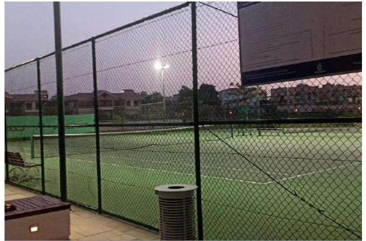
Tennis courts – fencing repairs and paint touchups in progress
