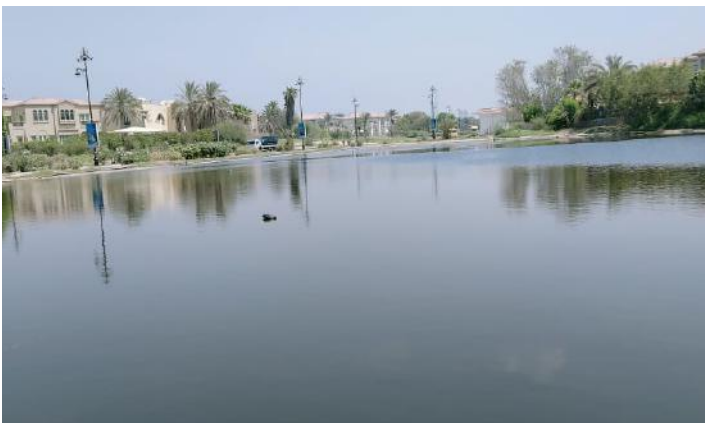
Installation of 8 subsurface diffusion aeration systems in the lake between Clusters 8 & 10. Location of aerators is indicated by black-coloured decorative ducks (for maintenance reasons).
