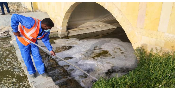
Ongoing clearance of screens and filters from debris, sediments and algae.
