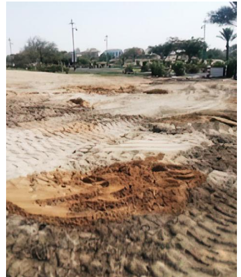
Fruit Farm - soil works completed between Clusters 19 & 20
