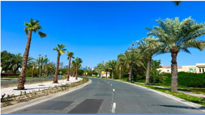
Centre median and right-of-way road works have been completed.
