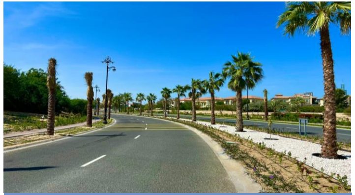
Landscaping enhancements have been completed along the main driveway.
