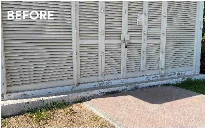
Jumeirah Islands has 38 substations that needed a face lift.
